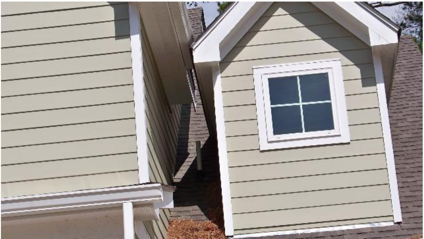
Roof dormer configuration at front
