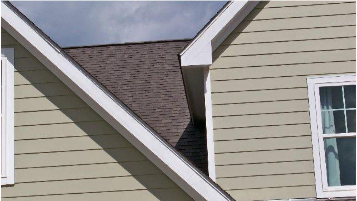
Roof dormer configuration at front
