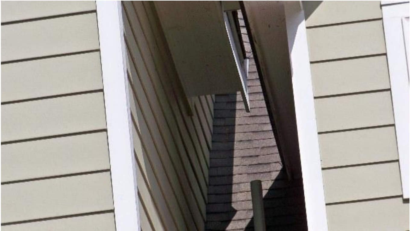
Roof dormer configuration at front
